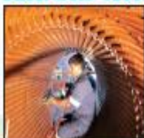
Core Scanning on 25 MW TG
